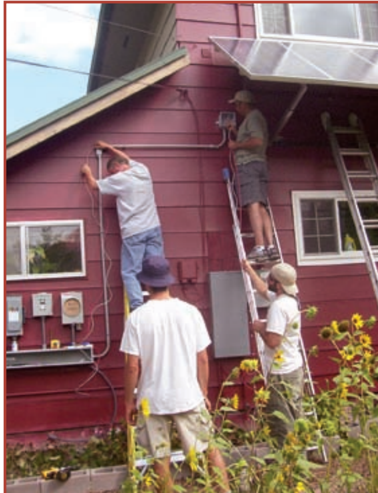
Running the DC wiring from the array to the disconnect.
